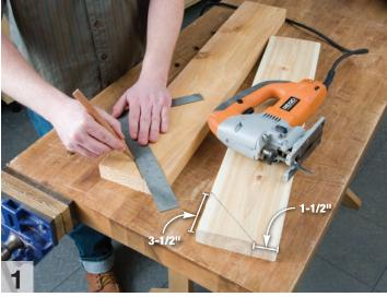
Mark the taper cut lines on the bench legs. Use a miter saw, jigsaw or handsaw to cut the tapers.
