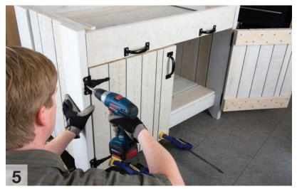
Position the hinges so that the bottom/top edge of the vertical plate is 1 in. from the bottom/top edge of the doors.
