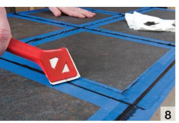
Fill the gaps between the tiles and around the perimeter with silicone caulk. Screed off the excess caulk with a caulk-smoothing tool or plastic putty knife.
